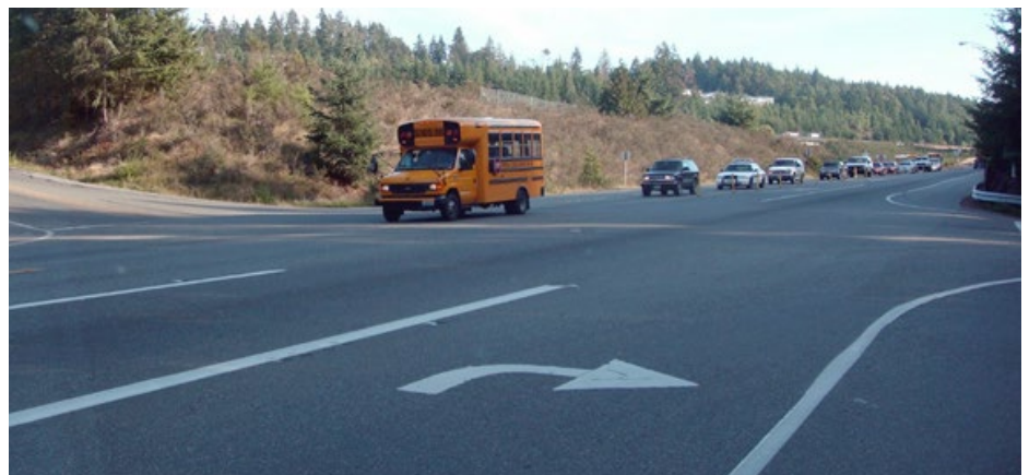
Example of a right-turn lane.
