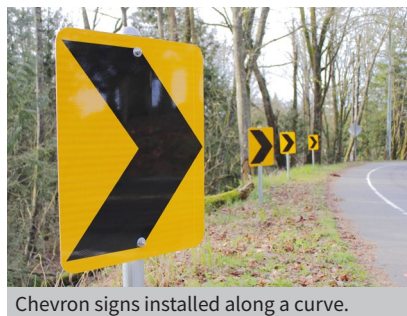
Chevron signs installed along a curve.
